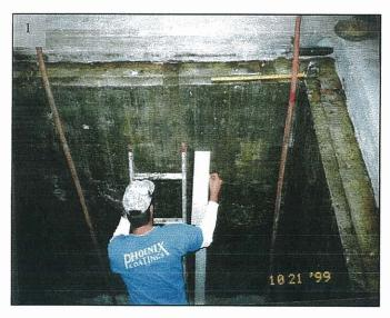
4" cap strips of 2 mil  $FluoroGrip^{TM}$  M treated on **two** sides and laminated with acrylic adhesive were used at the corners of the chute and where two sections of  $FluoroGrip^{TM}$  M were butted against each other.
