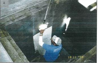
A roller was used to help facilitate bonding between the acrylic pressure sensitive adhesive and the primed concrete surface. Adhesive bonds immediately with maximum adhesion in 24 hours.
