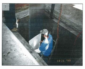
24" rolls of 10 mil *FluoroGrip™* M treated on one side (will not overlap) and laminated with acrylic adhesive were used to coat the 140 square foot surface. The cap strips were placed underneath the 24" film to reinforce the butt seams.
