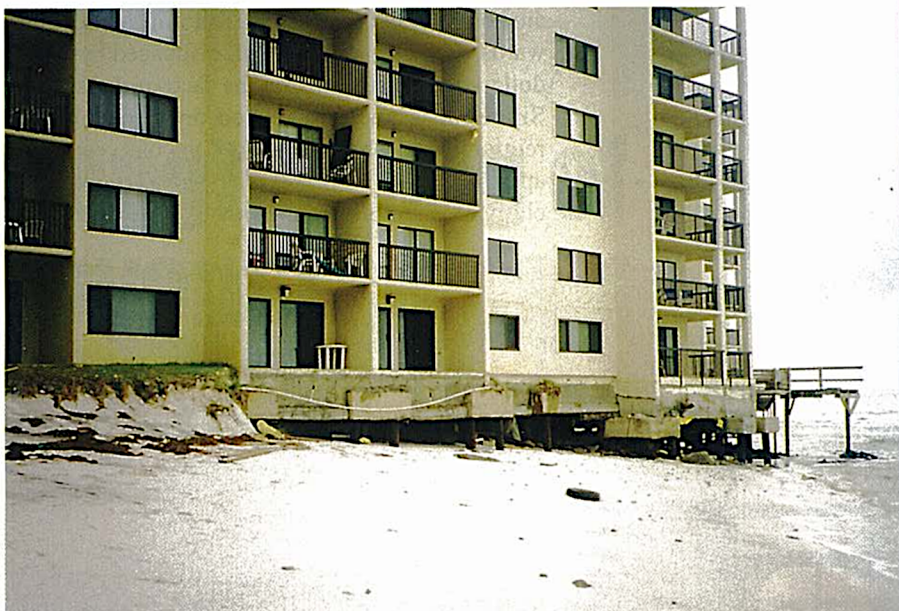
Figure 3: After Hurricane Georges, the turned down beams on the edge of the first floor slabs closed the gap between pile caps and saved the slabs on grade from collapsing
