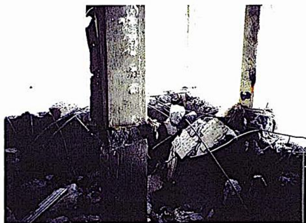
Figure 1: One of the "too tall" columns after Hurricane Opal and the remains of the first floor slab
