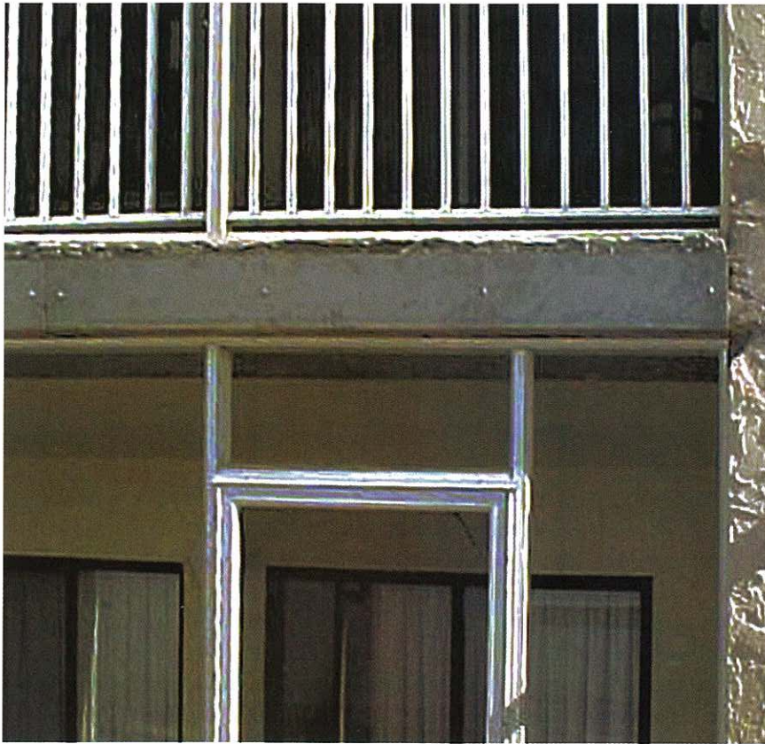
During concrete restoration at Holiday Surf and Racquet Club.
